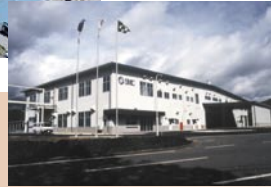
■ Tohno Factory (Iwate Prf.) Total Land Area: 79,428m 2 Floor Space: 10,737m 2
